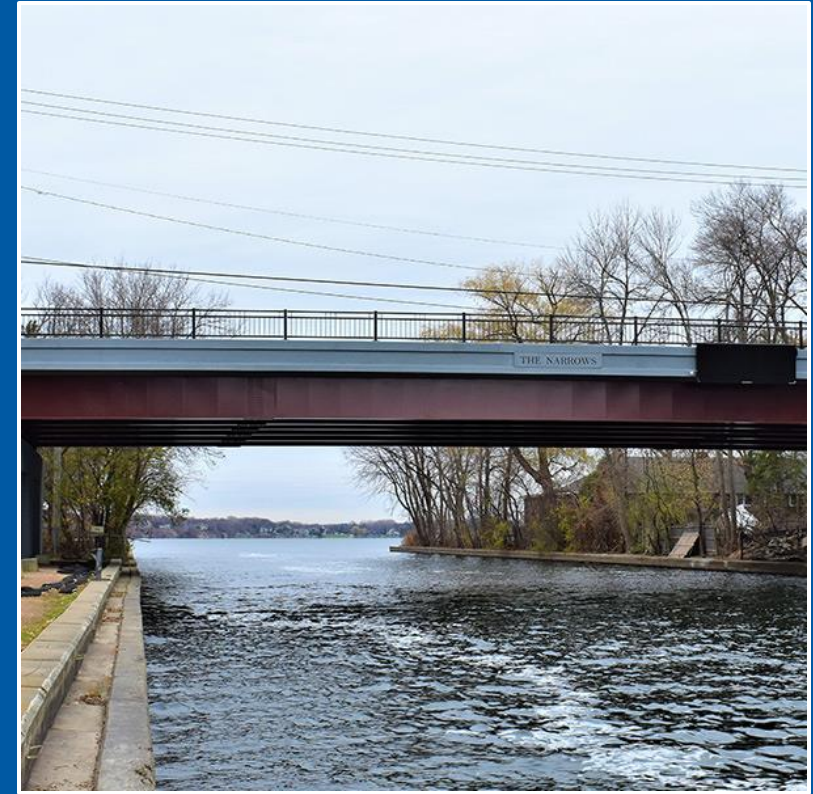
Narrows Bridge reconstruction
