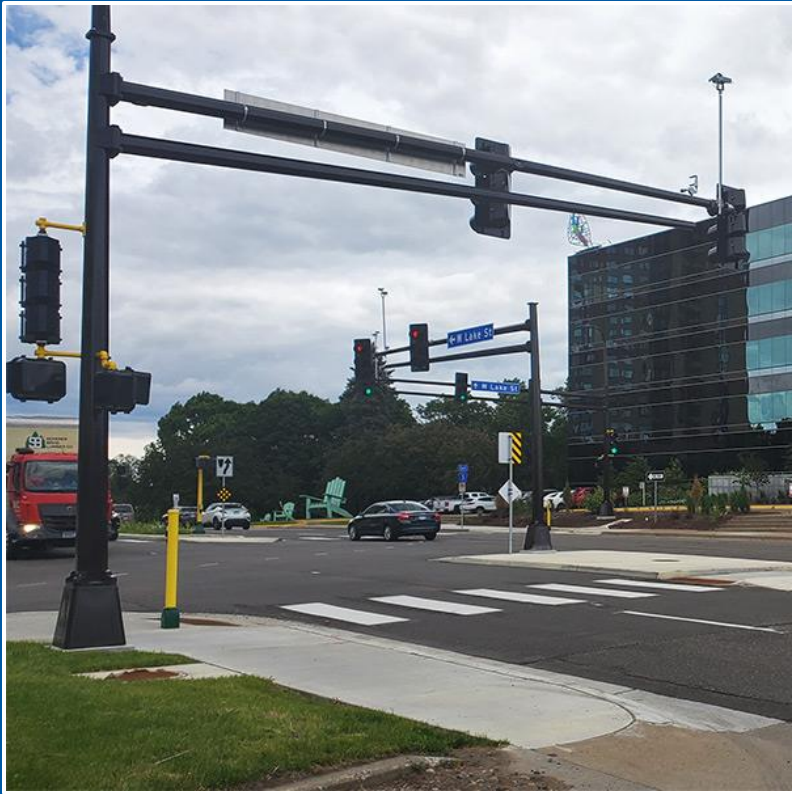
Lake Street and Excelsior Boulevard intersection improvements
