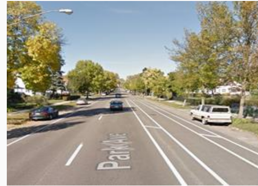
Bike lane striping
