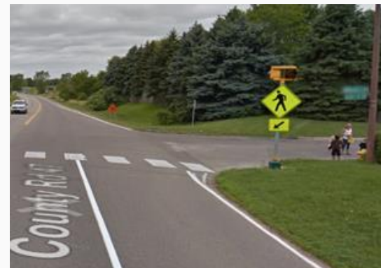
Rectangular rapid flashing beacon (RRFB)
