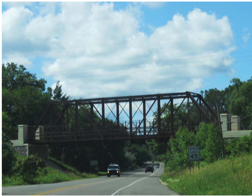
Before View Looking Northwest at the Luce Line Bridge Gateway
