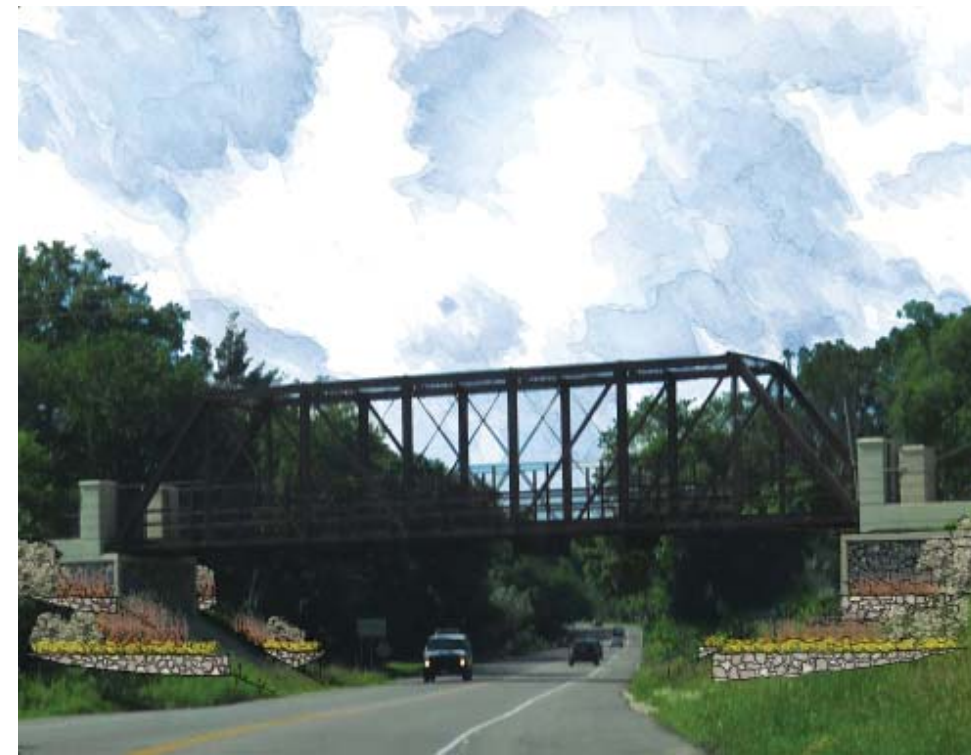
After View Looking Northwest at the Luce Line Bridge Gateway
