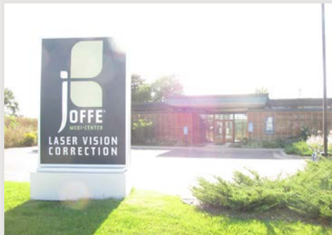
Existing office adjacent to future station
