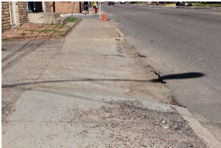
Figure 40. Example of Deteriorated Curb Face
