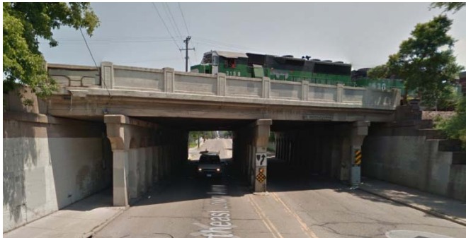
Figure 7. Railroad Viaduct Lacks Pedestrian Scale Lighting
