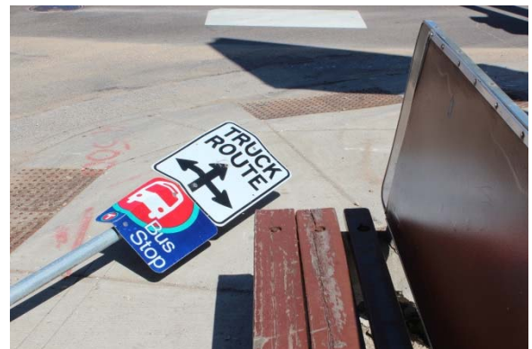
Figure 8. Bus Stop sign Knocked Over by Turning Truck
