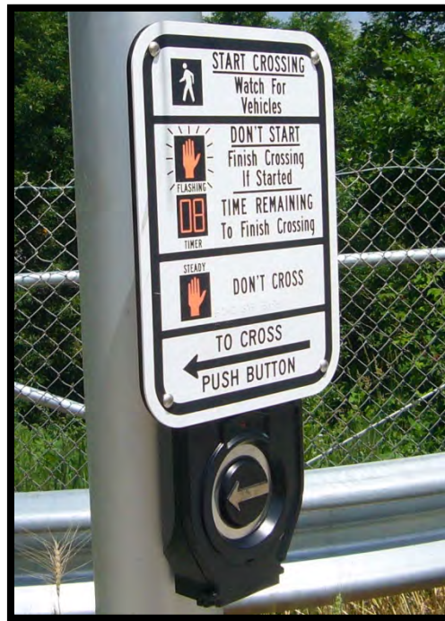
Figure C-5 Traffic Signal Pedestrian Phase
