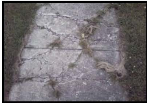
Cracking
