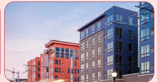
Fig. 11: Multi-family housing, particularly near stations, is needed
