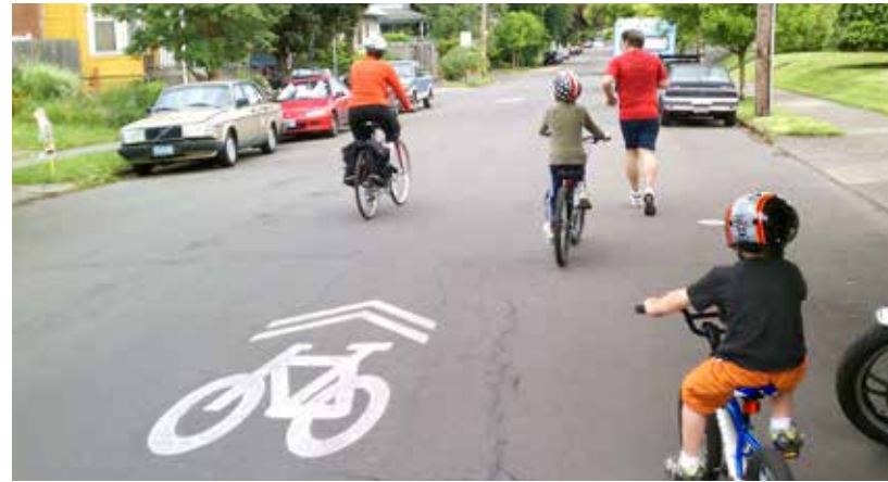
This is a bicycle boulevard in Portland, OR. Pavement markings indicate that the roadway is a shared street. A bicycle boulevard is recommended for Hubbard Avenue.
