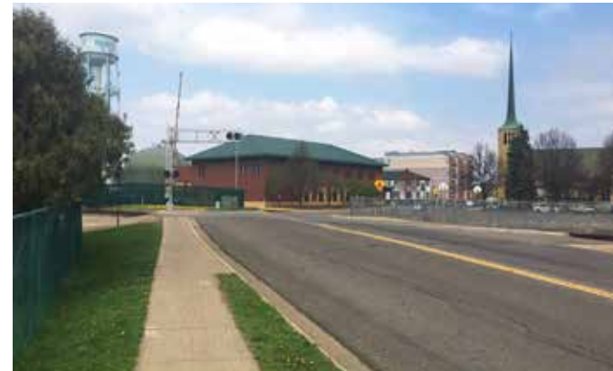
Existing Rail Crossing at 41st Avenue North
