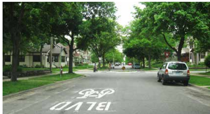
This is a bike boulevard on 17th Avenue South in Minneapolis. The neighborhood roundabout helps slow traffic, making the street more comfortable for people biking.
