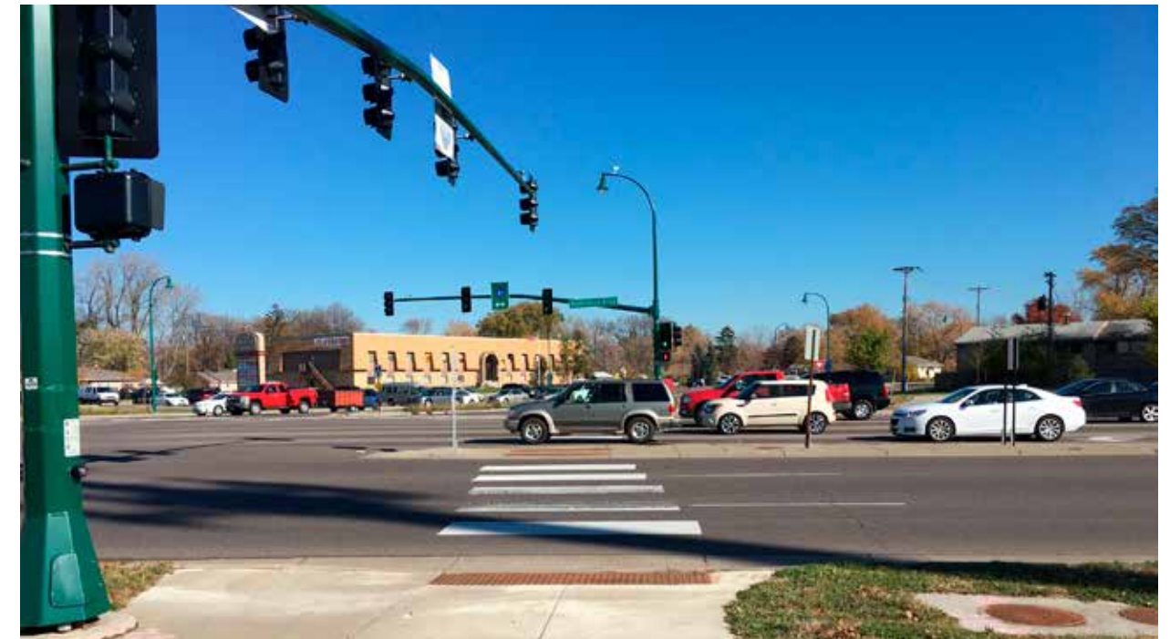
INTERSECTION OF BASS LAKE ROAD AND COUNTY ROAD 81
