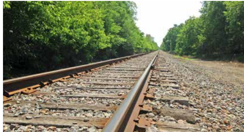
RAIL CORRIDOR The area along the rail will be reconfigured and landscaped. Views from the station into Becker Park will create a vision for riders of Crystal as a destination.
