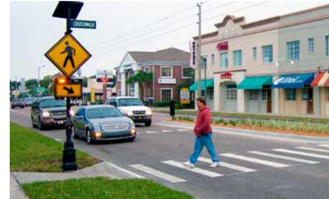
Rectangular Rapid Flashing Beacons (RRFB) and Pedestrian Crossing Signage
