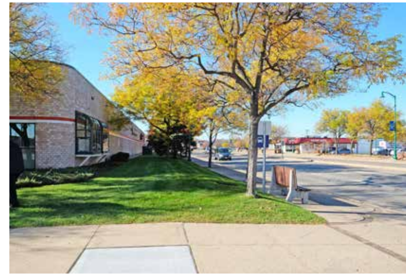
Bass Lake Road existing conditions
