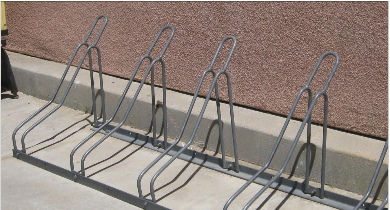
**Discouraged —Toaster:** These and other designs that support a wheel but not the frame may damage wheels and do not allow locking to the bike frame. *Credit: bikingintheav.com*
