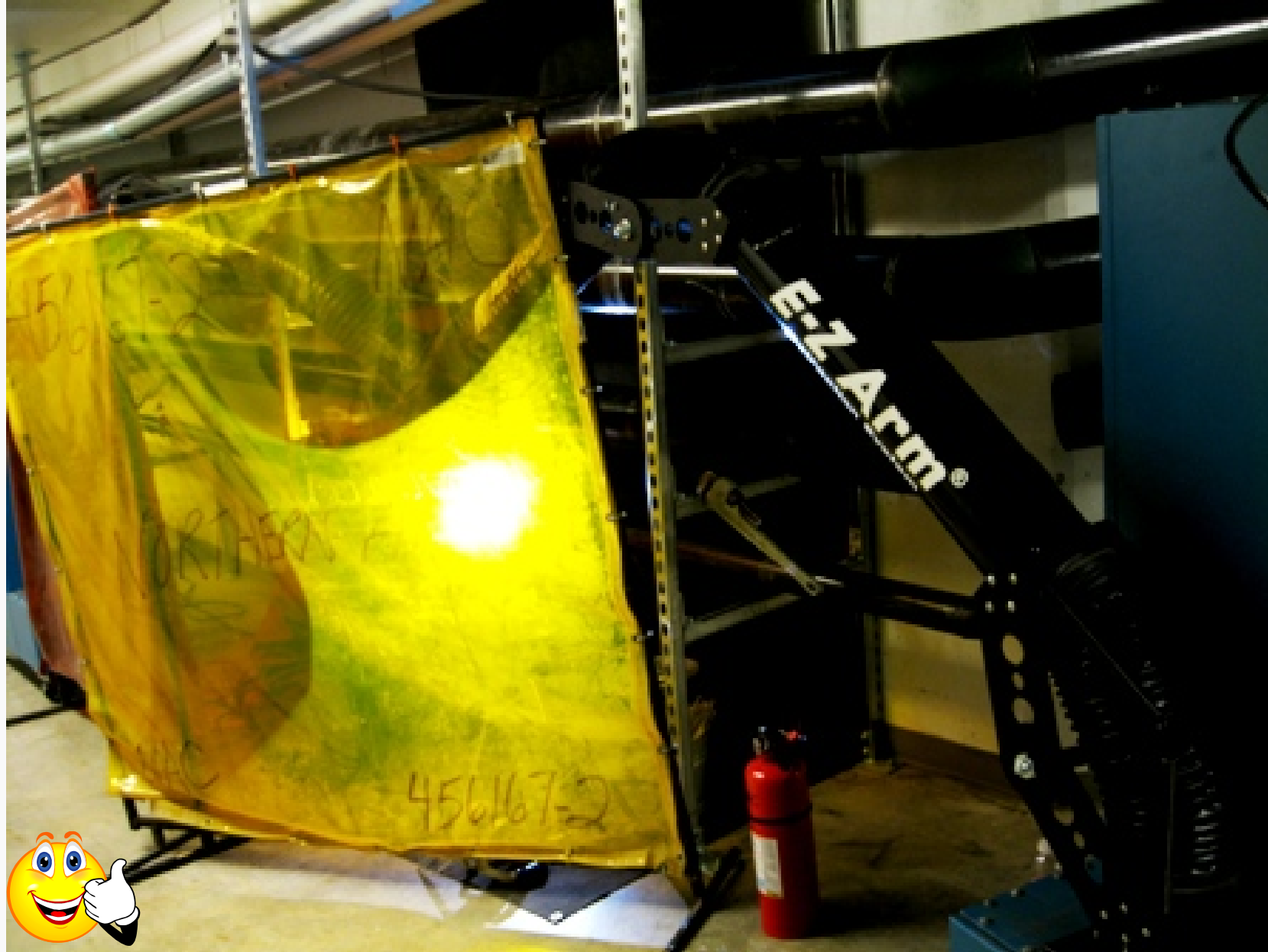
Note fire extinguisher and “smoke eater” in this welding operation.
