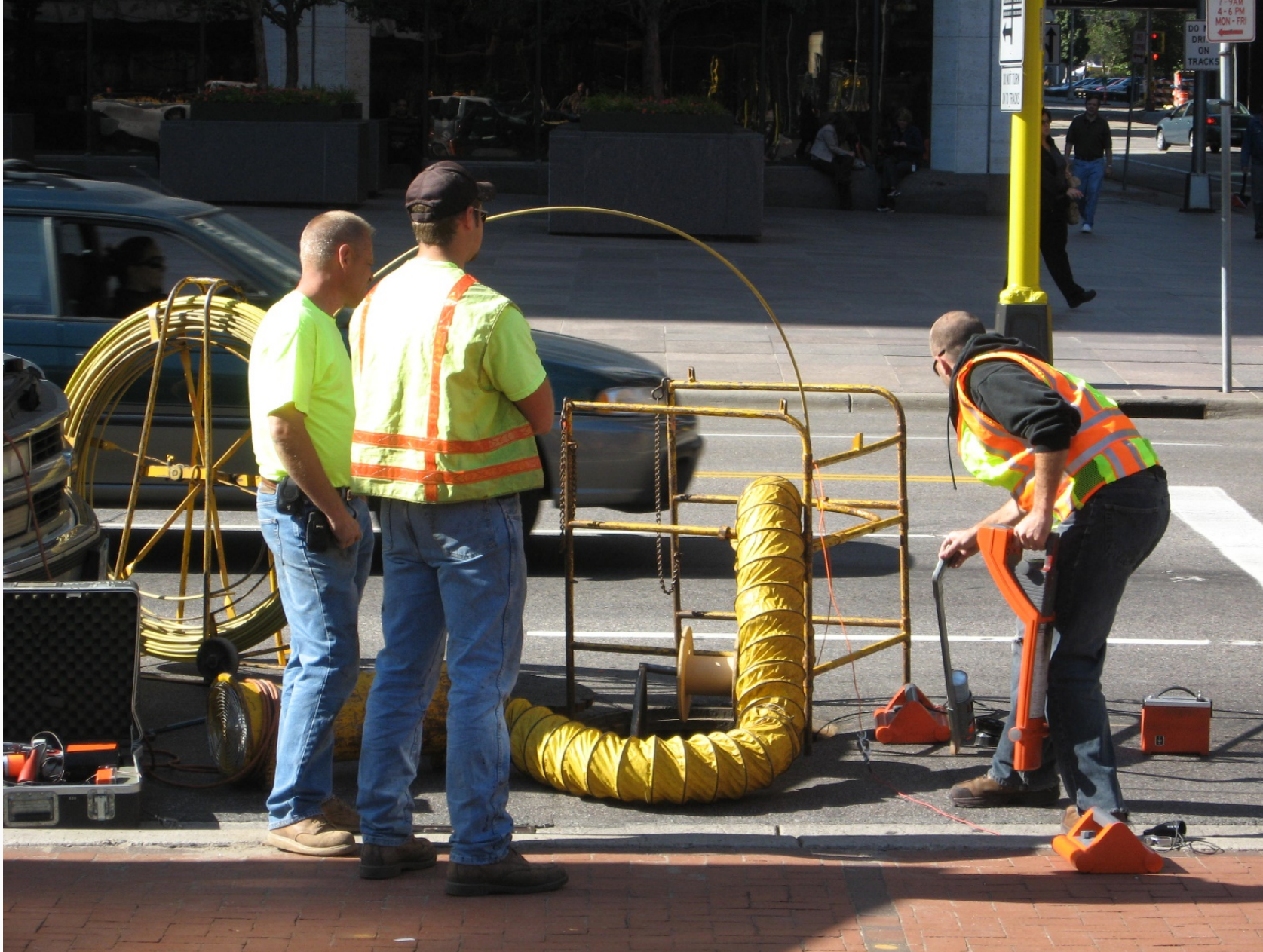
Work in confined spaces requires considerable equipment and extensive worker training.
