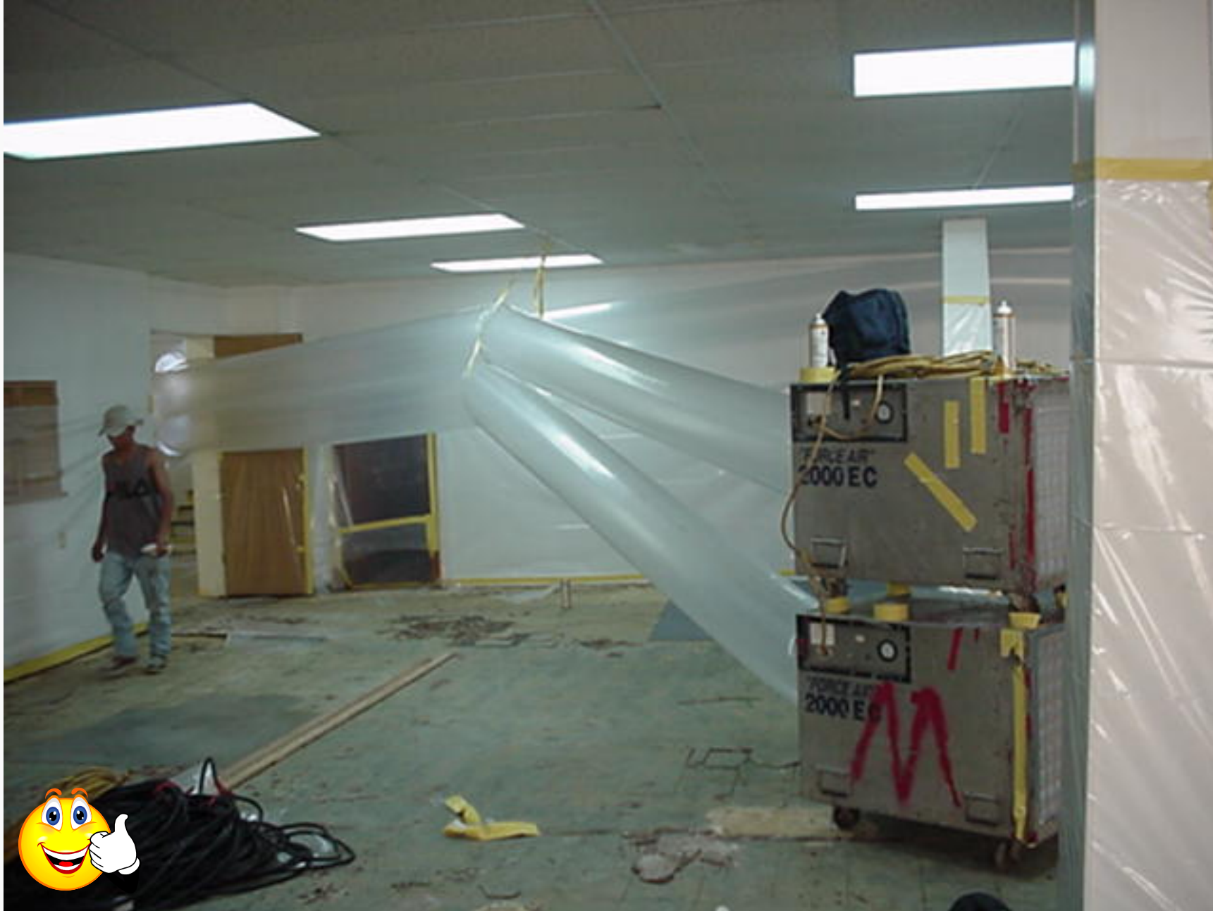
Use filtering fans with exhaust tubes directed to the outdoors to control dust and odors.
