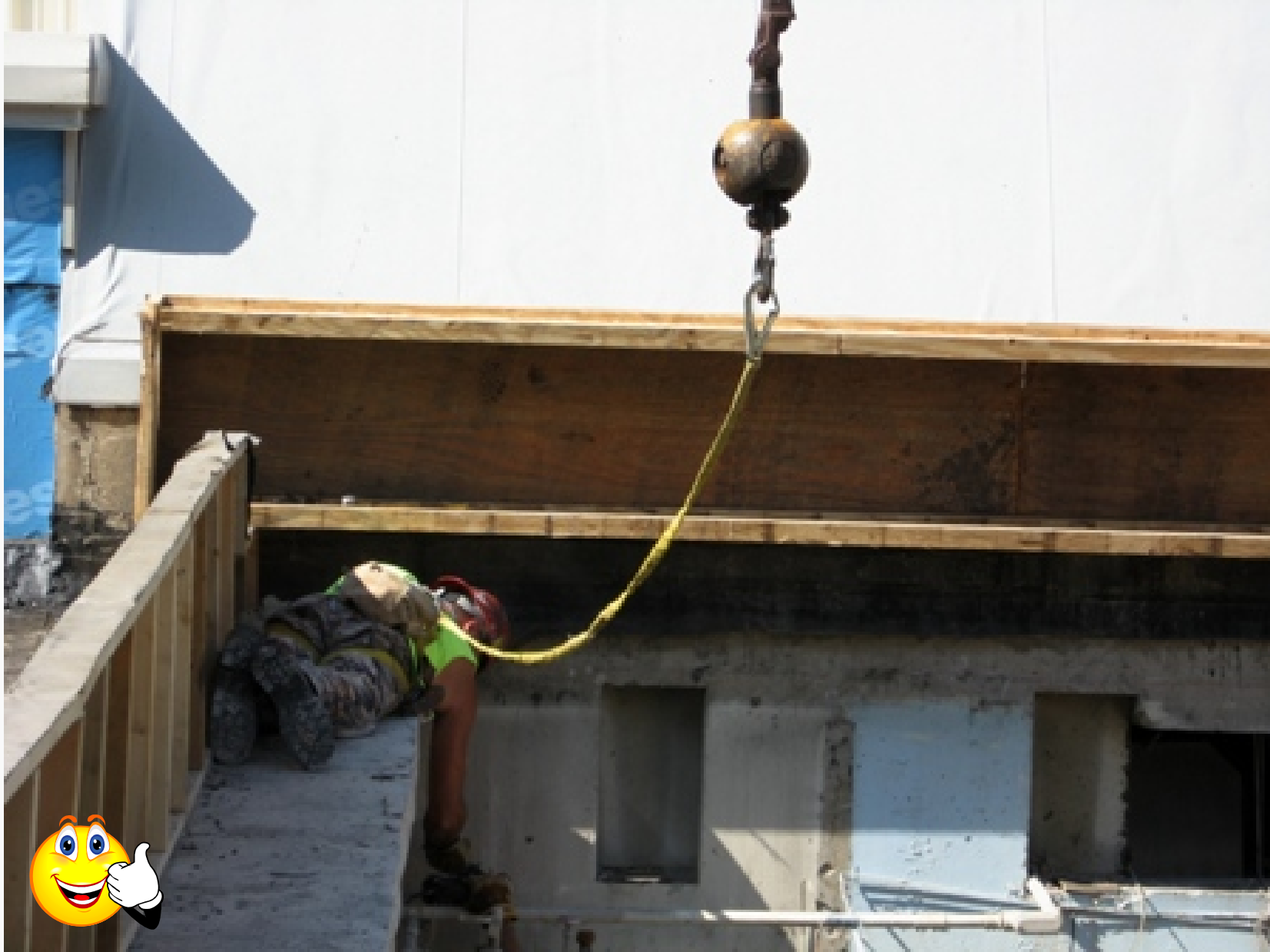
Construction worker using crane ball for fall protection anchor.
