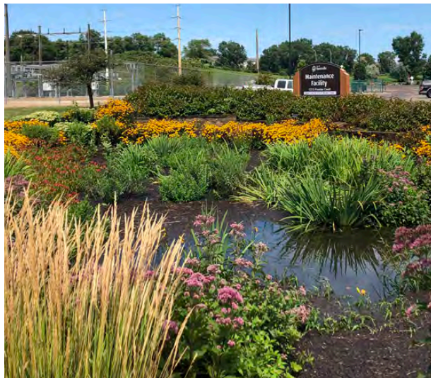
Biofiltration basins have the capacity to store stormwater as they treat it. Green stormwater systems create native habitat, increase the tree canopy, and improve water quality.
