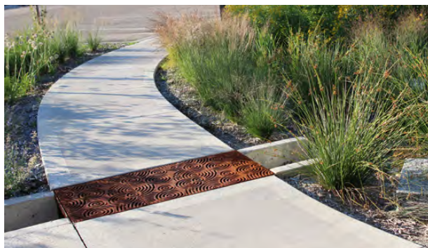
Stormwater can be conveyed from one area to another for treatment through artistic elements like this grate.
