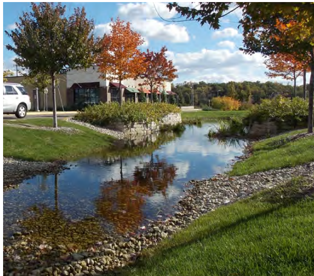
ABOVE Using natural drainage systems like this bioretention basin helps remove pollutants and reduce stress on county and municipal storm sewer systems.
