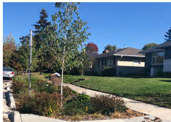
ABOVE Using natural drainage systems like this bioretention basin helps remove pollutants and reduce stress on county and municipal storm sewer systems.
