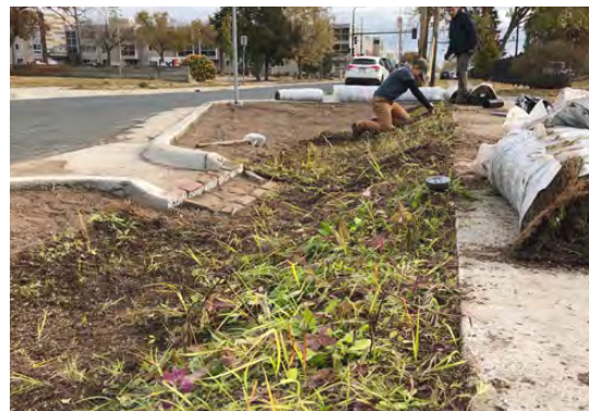
Blankets of pre-grown vegetation are rolled onto the site for instant native plant cover.
