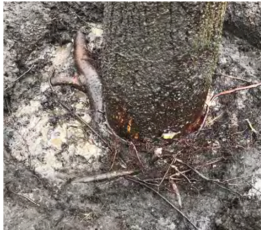
Stem girdling roots around the base of a tree threaten its health and longevity.
