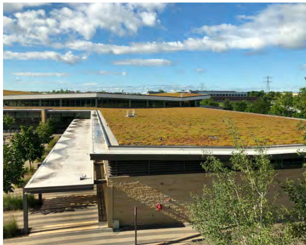
Green roofs reduce runoff by storing and absorbing rainwater where it falls, while also filtering excess water as it drains through the plant layer.
