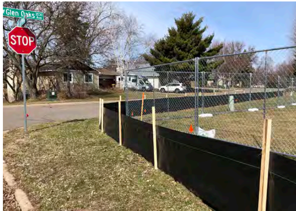
Silt fence perimeter protection installed around project site before construction
