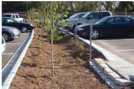
Design stormwater BMPs to be landscape amenities such as this parking lot rainwater garden whose trees will shade the parking lot.
