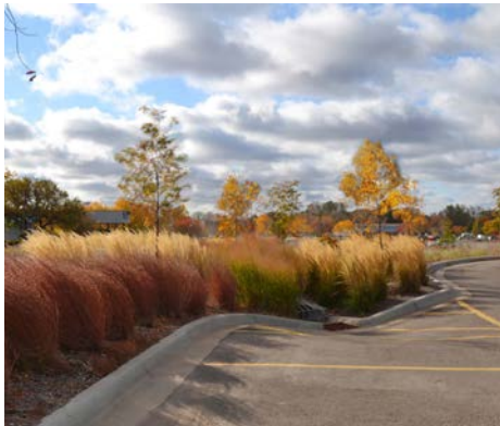
Incorporate stormwater bioretention basins where possible, such as along parking lots to enhance ecological function by capturing stormwater for the benefit of plants, local streams and groundwater.
