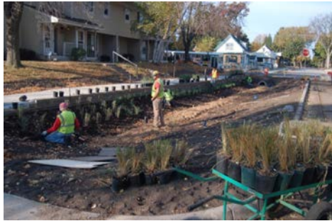
Routine inspections during planting provides opportunities for directing crews and preventing problems such as planting too deeply or supplying the wrong plants.
