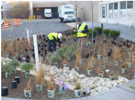
Routine inspections during planting provides opportunities for directing crews and preventing problems such as planting too deeply or supplying the wrong plants.
