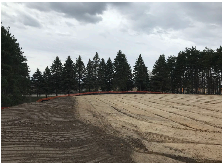
Tree protection at new Medical Examiners facility during construction
