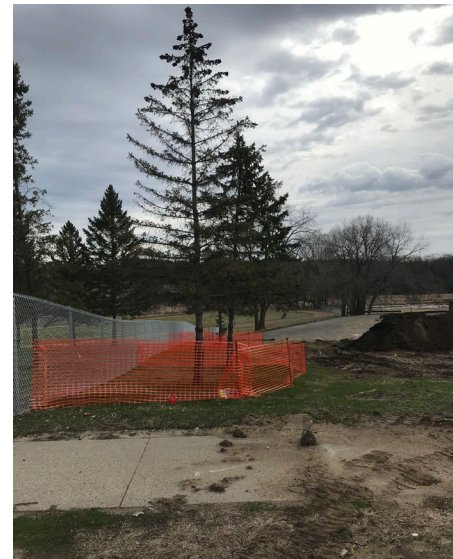
Tree protection at new Medical Examiners facility during construction
