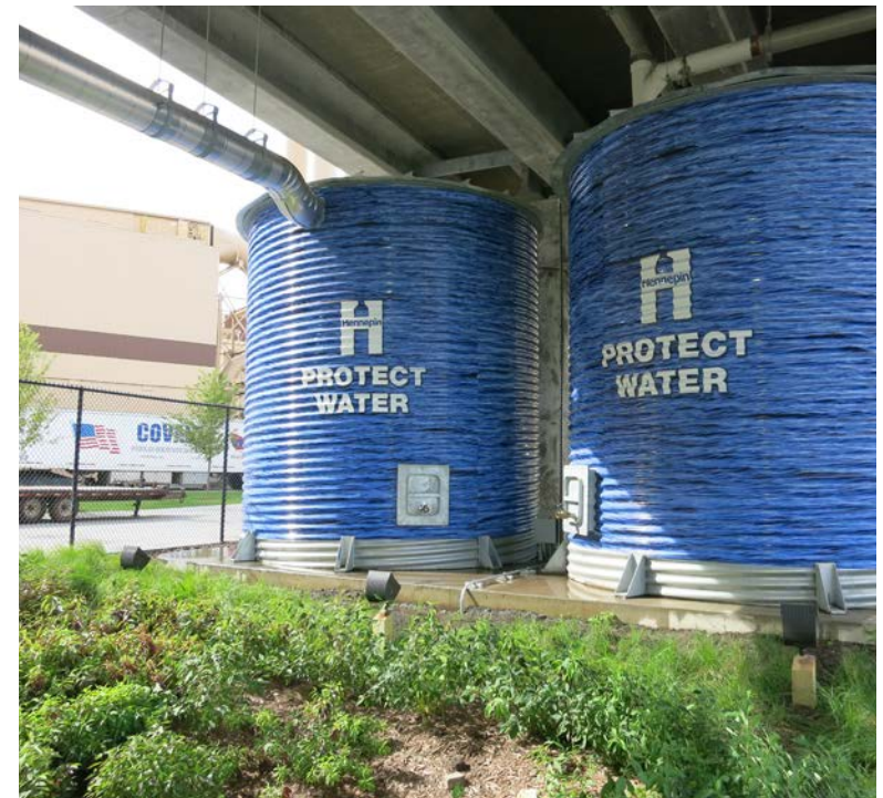
Target Field Station includes a variety of features, including these cisterns and bio swale that capture and filter approximately three million gallons of rainwater and snow annually.
