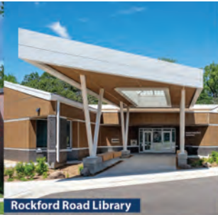
Rockford Road Library
